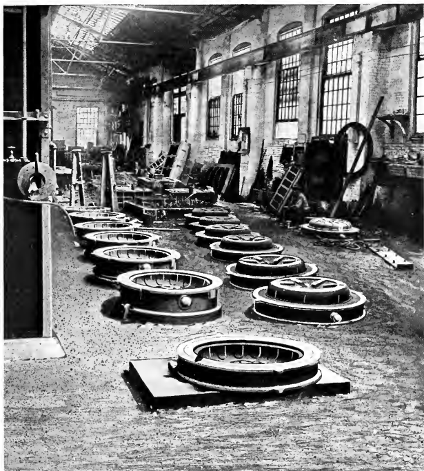
Fig. 76. A floor of Generator End Frame Moulds made on the Plain Jolt Machine shown in the foreground, at the plant of THE WESTINGHOUSE ELECTRIC & MFG. CO. Cleveland, Ohio, U. S. A.
